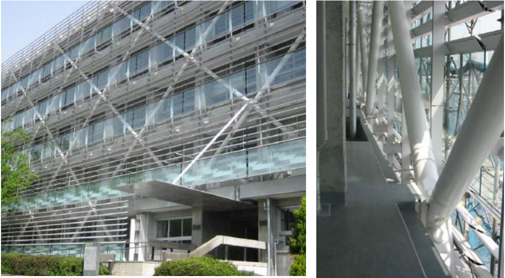
Figure 2.7. Engineered steel exoskeleton in the Midorigaoka-1st building [25]
