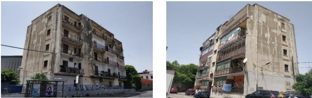
Figure 7.2. Case study building located in the city of Catania (Southern Italy)
